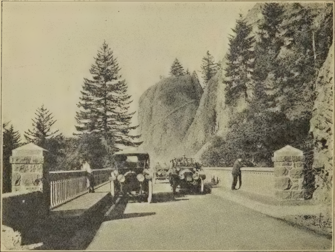
BRIDGE ON THE COLUMBIA HIGHWAY, OREGON
